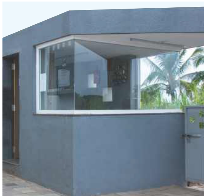
GLASS TO GLASS JOINT WINDOW
